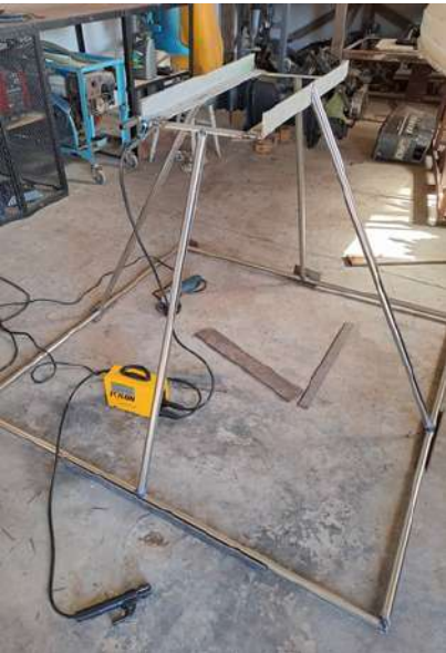
We welded a casing.
