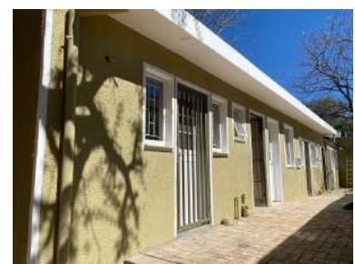
KFF's new flexible spaces in an office within The Hub premises.
